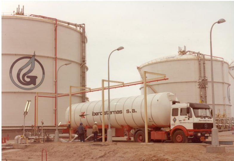
Barcelona LNG truck loading 26 February 1982
